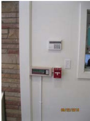
FA Remote Annunciator/Pull Station
