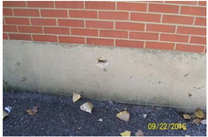
Spalling to be Repaired
