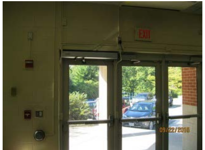
Door Contacts/Exit Signs/FA Devices
