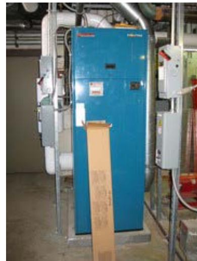
Gas Fired Boiler
