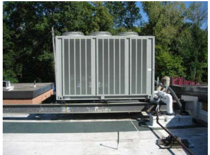
Air Cooled Condenser
